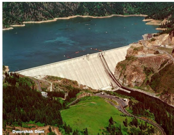
Fig 5.2 Gravity dam - Dworshak Dam
