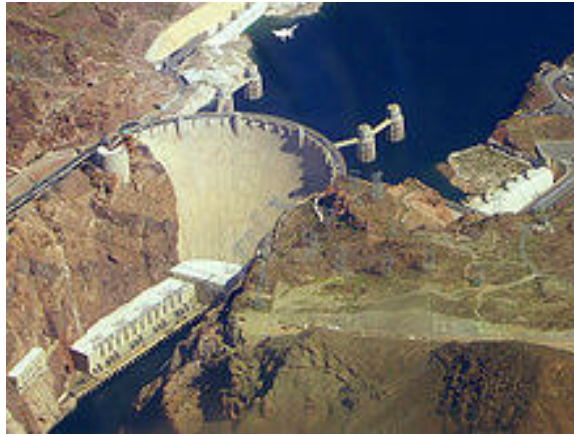
Fig. 5.1: Arch-Gravity Hoover Dam
